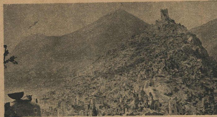
Not a building remained intact.
