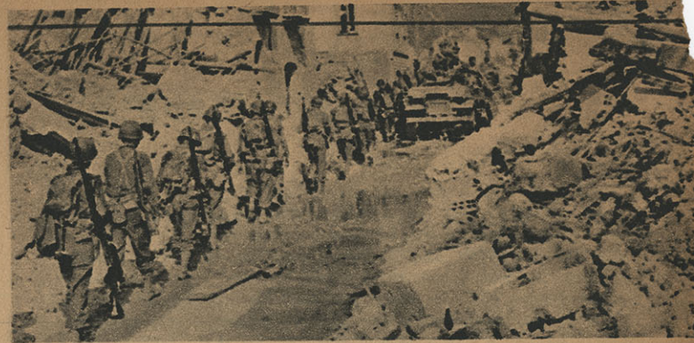
Reinforcements kept coming.
